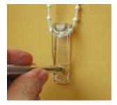
Step 3 - Mark out the hole. If fixing to wall, drill the hold to the depth of the screw provided using a 5.5mm drill bit and place wall plug into hole.
