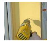
Step 4 - If fixing to wall, drill the hold to the depth of the screw provided using a 5.5mm drill bit and place wall plug into hole.
