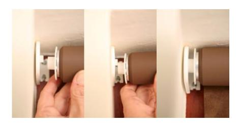
12. Now insert the roller tube into the brackets. First put in the plunger end and again push it slightly to depress the plunger enough so that you are able to insert the sidewinder/ control end. When inserting the control side you will see that the end of the blind has a star- shaped hole, which makes it possible to mount the blind in different positions.
